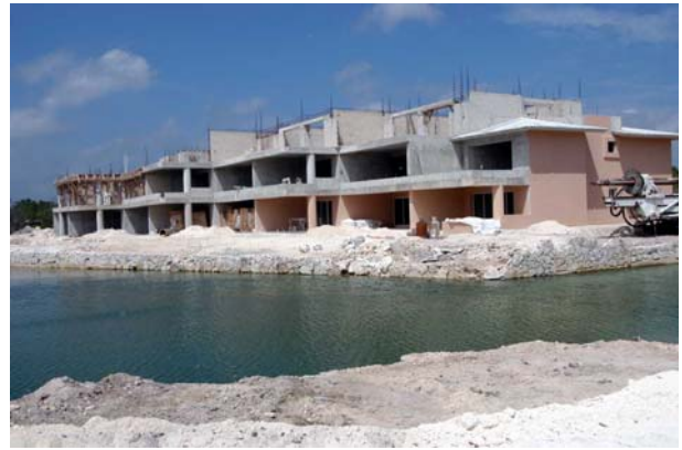
Figure 9: (top) Temporary coastal spring through caprock fracture on beach in Playa del Carmen, after Hurricane Wilma. (bottom) "Waterfront development" in Puerto Aventuras.
